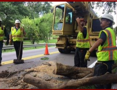
Road & Bridge 4 Crew Clearing Debris
