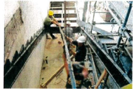
Installing the staircase. (photo by Ross Crabtree)
