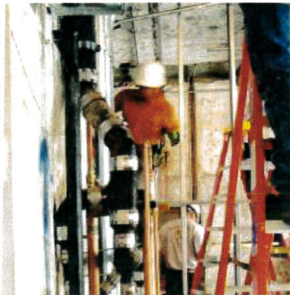
Workers roughing in a wall. (photo by Ross Crabtree)
