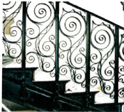
Detail of the staircase. (photo by Ross Crabtree)
