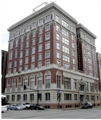
Dallas County Records Building Complex
