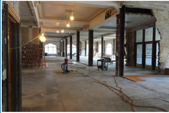
Records Building Post-Demolition Phase
