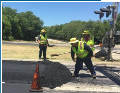
Road & Bridge 4 Crew Spreading Asphalt
