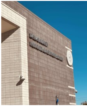
Top: Dallas County's new Mesquite Government Center
